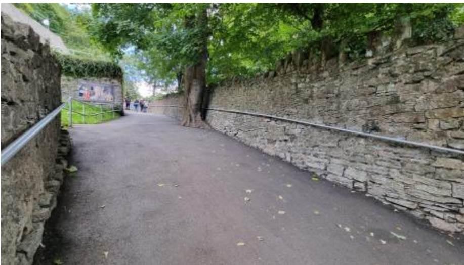
Photo shows the steep pathway leading to the main entrance. There is a handrail to the right.
